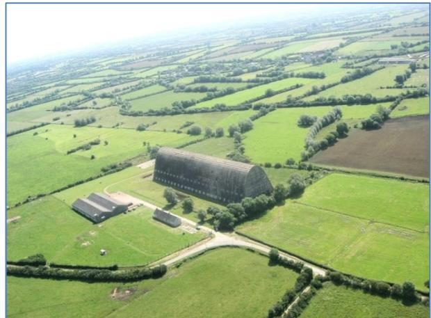
It is a remarkable work of human engineering which is entirely made up of reinforced concrete, including cover and structure: its higher section has a geometry of a reversed "catenary curve". Built by Etablissements Fourré and Rhodes (now in the EIFFAGE Group), it was fully completed in 1920.
